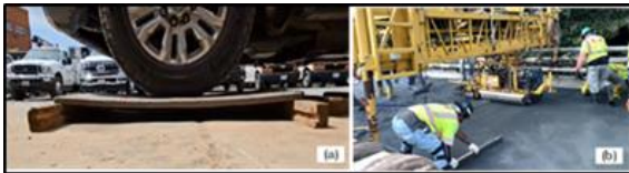
Figure 2. A 1-inch Thick Ultra-High-Performance Concrete (UHPC) (Burgess, 2024) and Cor-Tuf UHPC Application on GW Memorial Bridge Project (Cor_Tuf, 2024)
